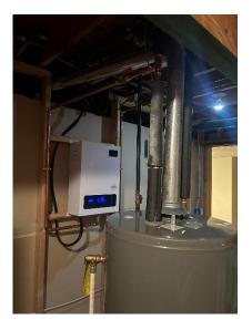
**Results:** The incoming water temperature was approximately 50 degrees. The tank heater was set at 115 – 120 degrees. The SIO 18 Pro was also set at 115 degrees... a 65 degree rise.
